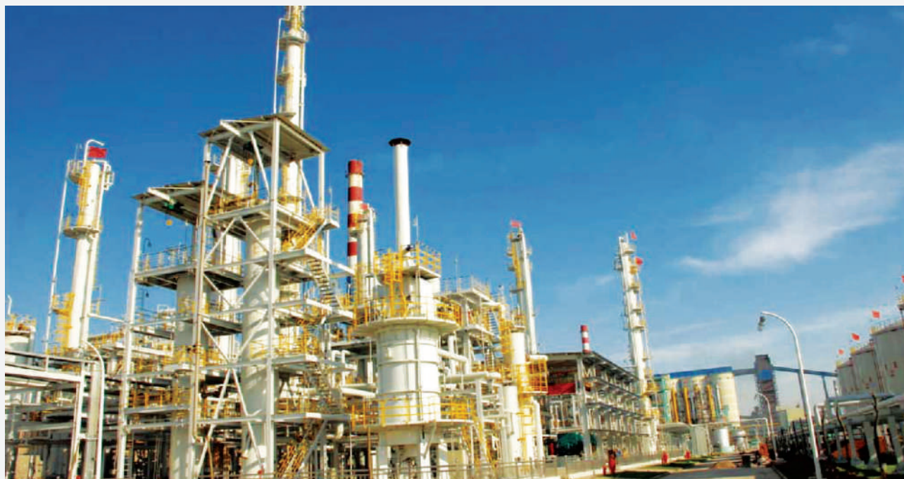
Sinopec Shanghai 3.9 mio tons/a high-pressure residue hydrogenation device
